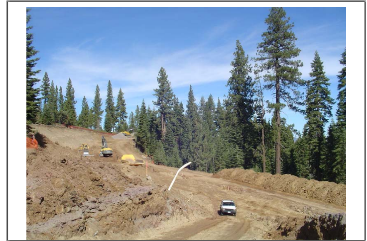
Highlands View Road Construction in Zone 3
