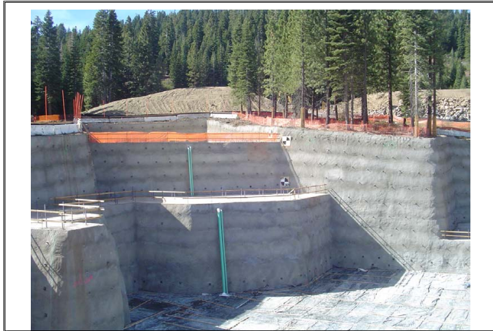
Ritz Carlton Hotel Foundation – Special Tax Zone 3
