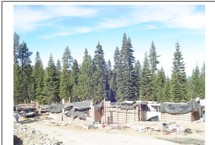
Trailside Townhomes Phase 1 – Special Tax Zone 3
