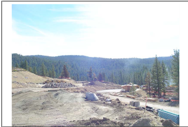
Intercept Parking Lots Under Construction
