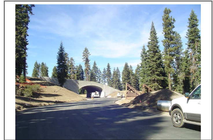
Highlands View Road & Village Express Road Tunnel/Skier Overpass
